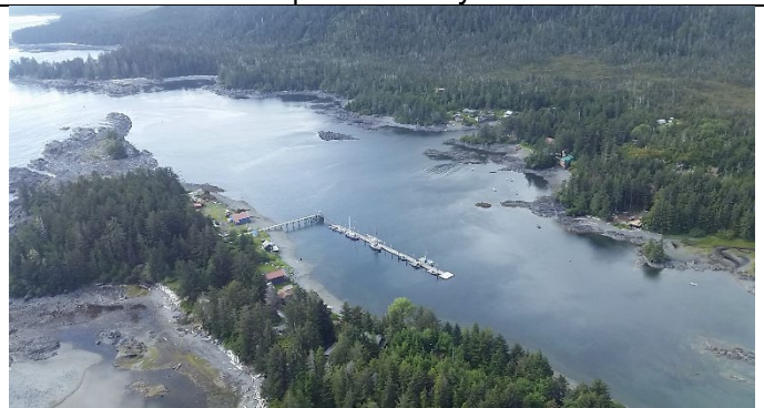
Port Alexander (AHP) 2024 DOT&PF | Community Off-Road
